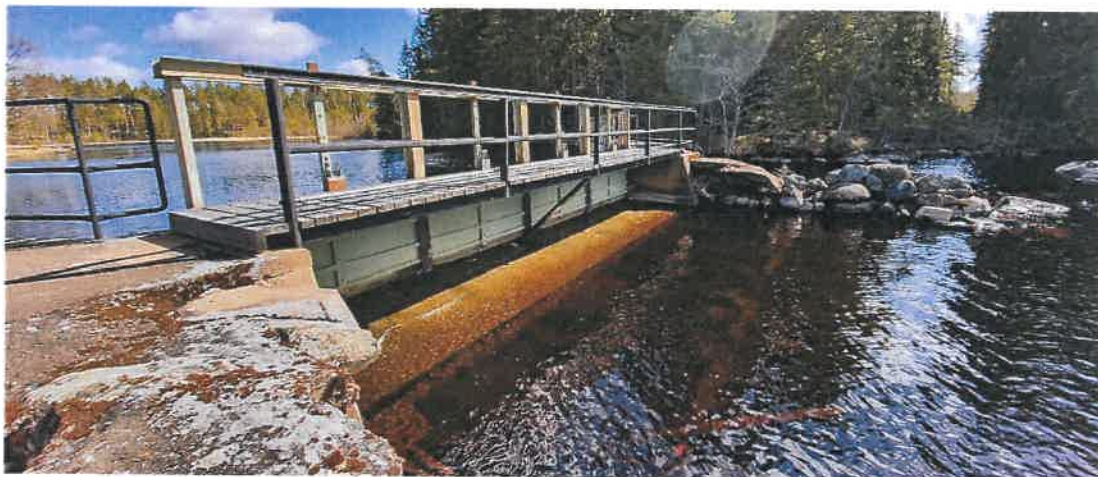
Figur 7. Sikfordsdammen, mellersta utskovet (Norconsult 2020-04-16)
