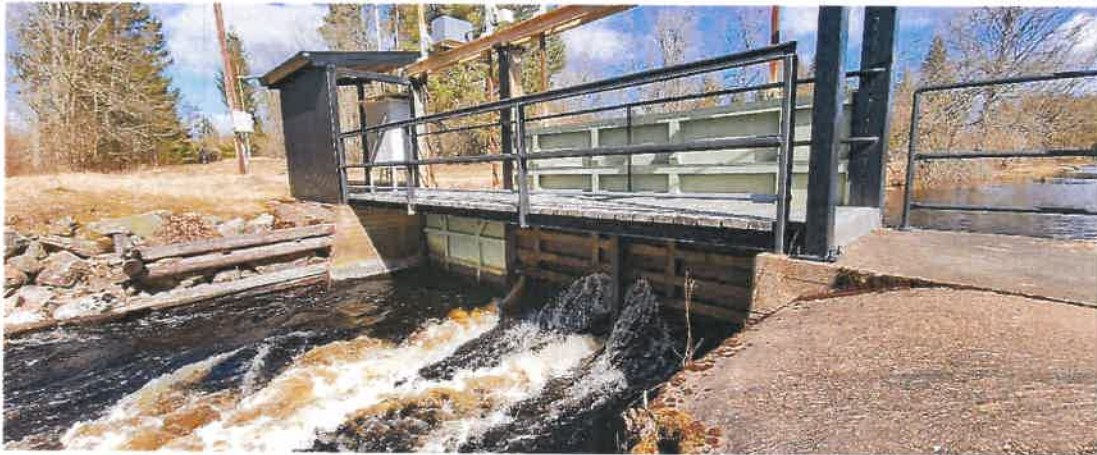
Figur 6. Sikfordsdammen, högra utskovet (Norconsult 2020-04-16)
